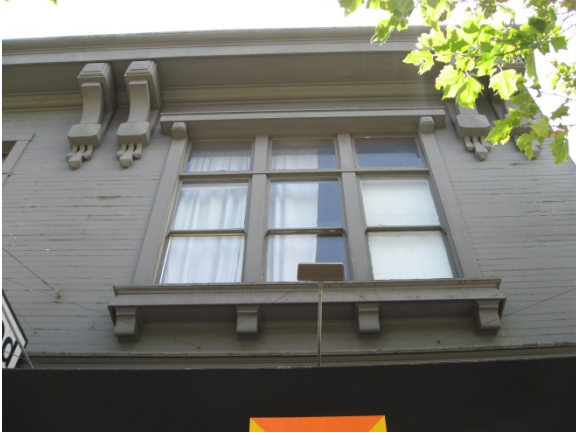
Detail of window and cornice
