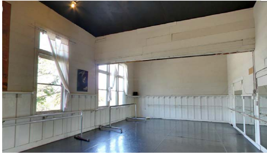
View east within Lodge Room No. 2. (Google Maps)
