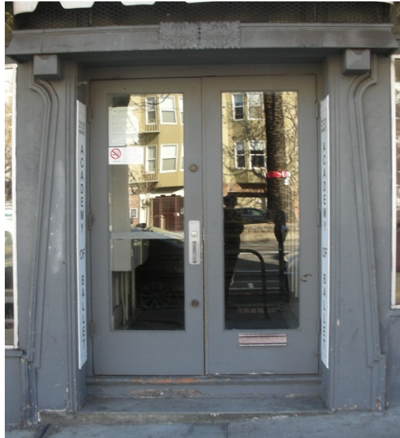
Center entry leading to Lodge Rooms
